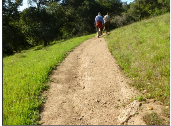
Images from left: Running slope with drainage channel parallel to the path of travel within the trail surface and cross slope running perpendicular to the path of travel. Both images are from Dwarf Oak Trail.
