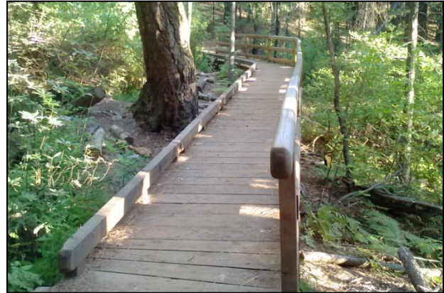
Images top row from left: Rock trail edging to define and hold trail edge and wooden wheel guide along boardwalk. Bottom row: Cable guide along the trail edge and a wooden guardrail section where there is a significant drop off from boardwalk surface to adjacent natural surface.
