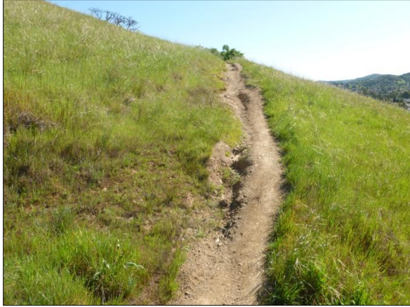
Images from left: Running slope with drainage channel parallel to the path of travel within the trail surface and cross slope running perpendicular to the path of travel. Both images are from Dwarf Oak Trail.
