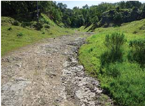
Figure 3.22 Competent shallow bedrock can minimize the amount of erosion, but at the same time can lead to an uneven road/trail surface.
