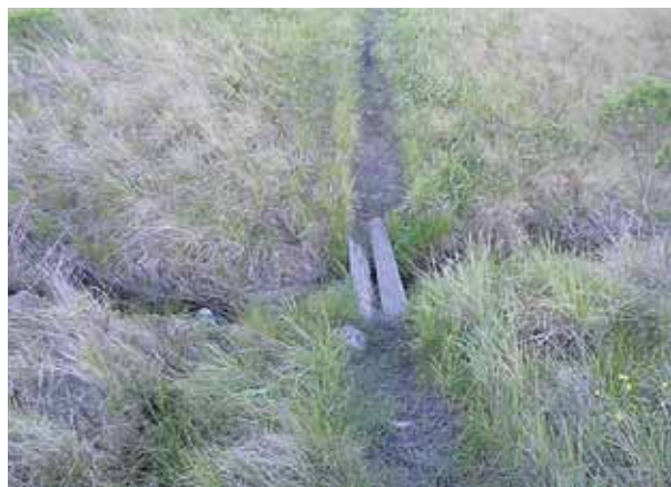
Figure 3.38 Informal puncheon over a small ephemeral watercourse.
