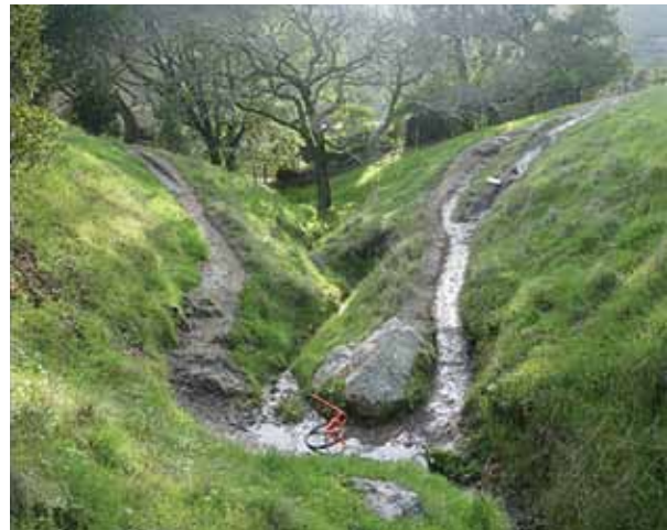
Figure 3.21 Erosion of seasonally wet and relatively weak cohesionless soils.
