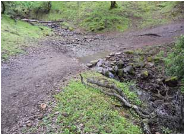
Figure 3.41 Rock ford on unsurfaced road. Ford constructed using native rock to armor outer road edge.
