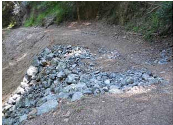
Figure 3.42 Rock ford on road-width trail.
