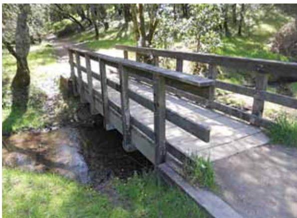
Figure 3.37 Functional wood foot bridge.
