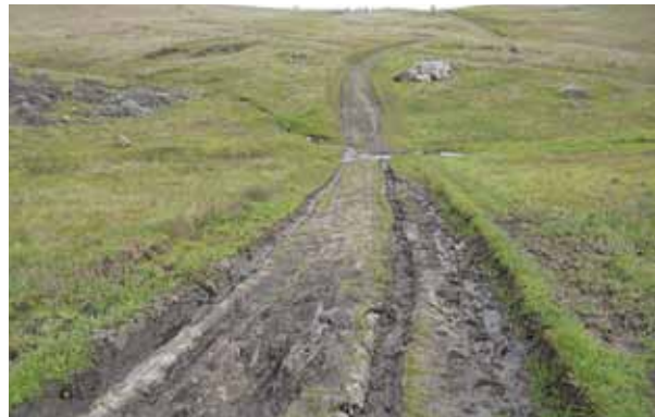
Figure 3.9 Short fall line road segment in seasonally wet and muddy soils. Road segment drains into watercourse and is responsible for chronic fine-grained sediment delivery.
