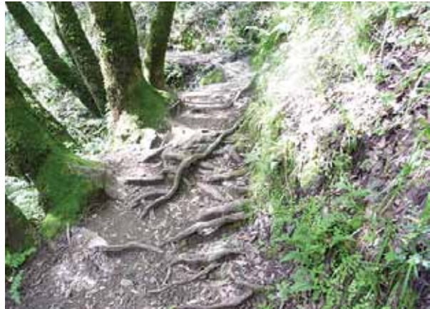
Figure 3.3 An example of poor tread condition.
