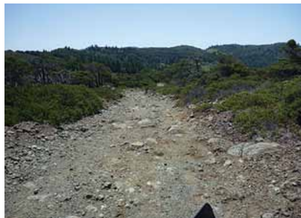
Figure 3.24 Irregular tread surface on ridgetop fire road routed through serpentinite bedrock.
