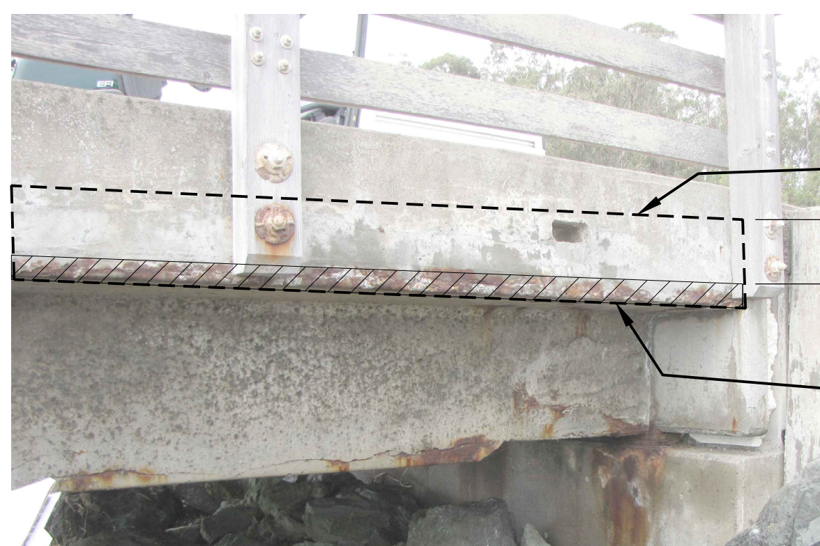
CORROSION AT EDGE OF TEE CURB REPAIR C2 S9
