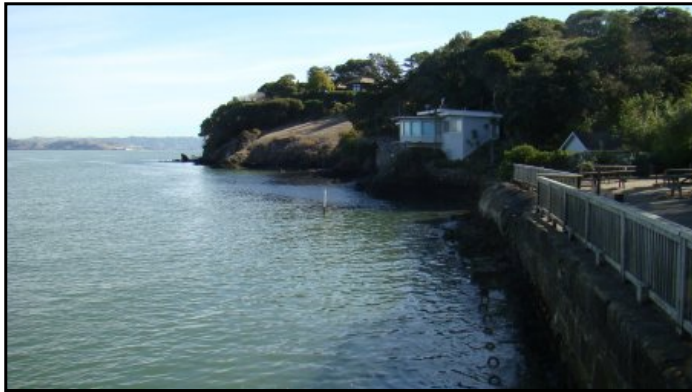
View of seawall; looking easterly
