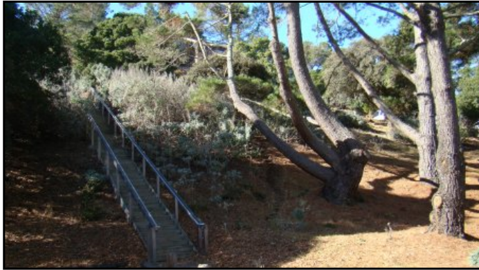
View of stairway leading to upper parking lot
