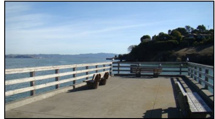
View of fishing pier; looking easterly
