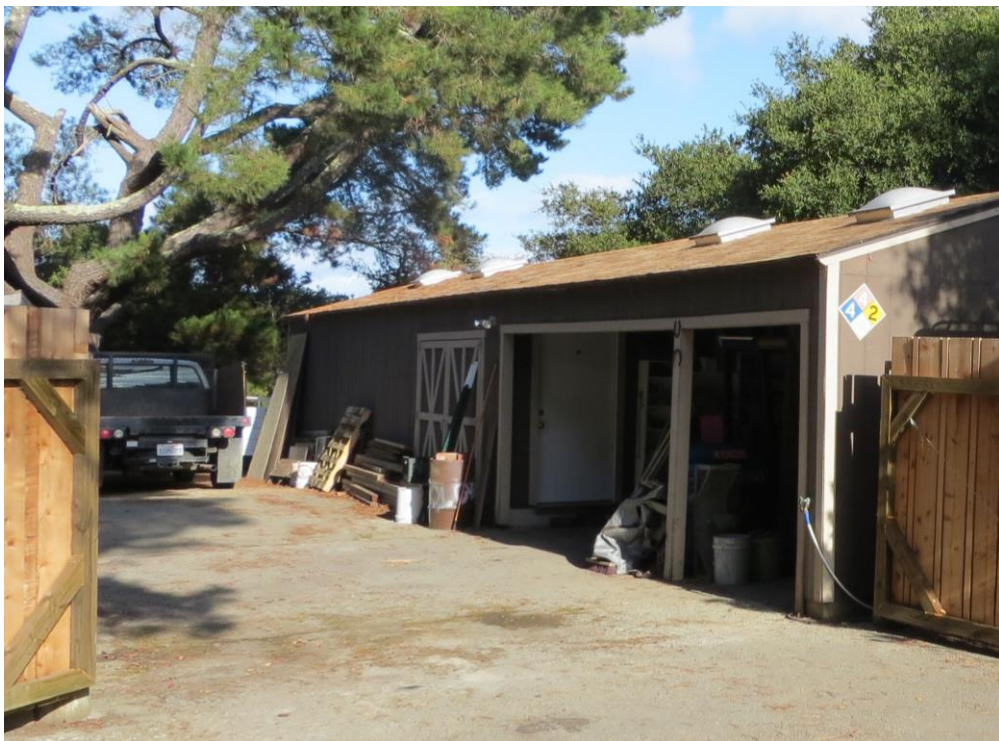
Figure 9. – View of maintenance shed from upper parking lot.
