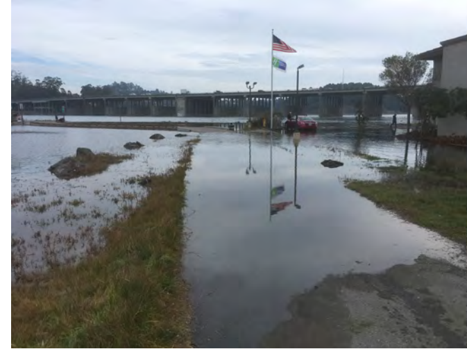
EDGE WEAR AT AREAS WITH KING TIDES
