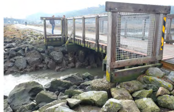
BRIDGE 2 - SOUTH BOTHIN MARSH CHANNEL
