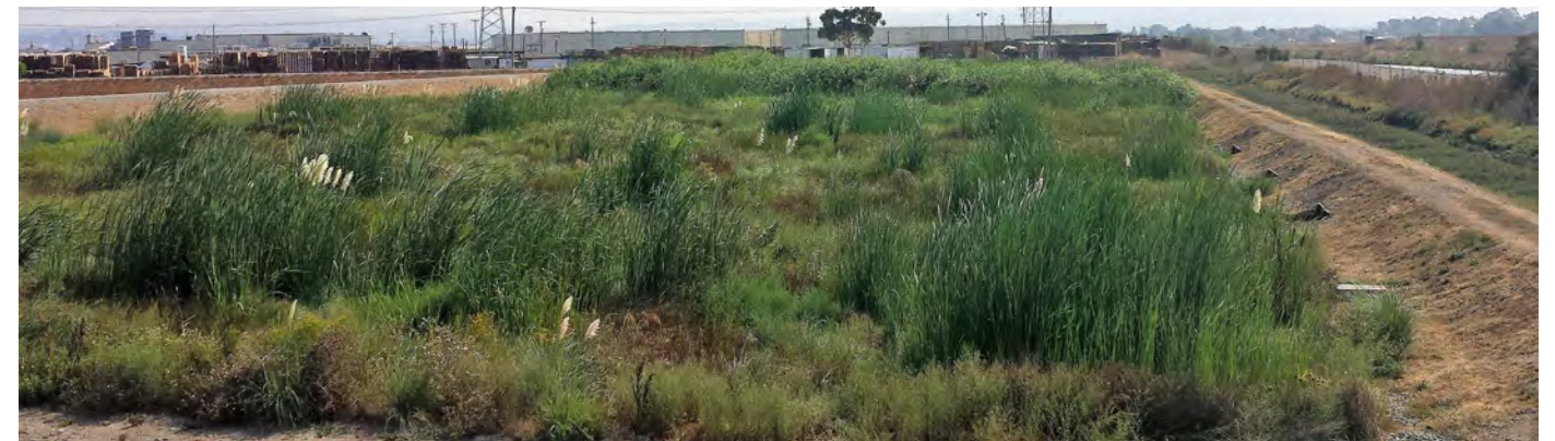
Horizontal Levee Project at Oro Loma Sanitary District, ESA, 2019.
