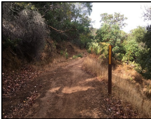
Photo 1: Landslide on Ponti Fire Road
