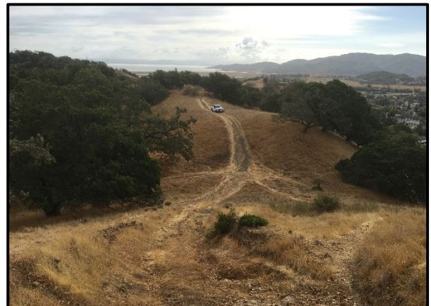
Photo 5: Steep Intersection looking east
